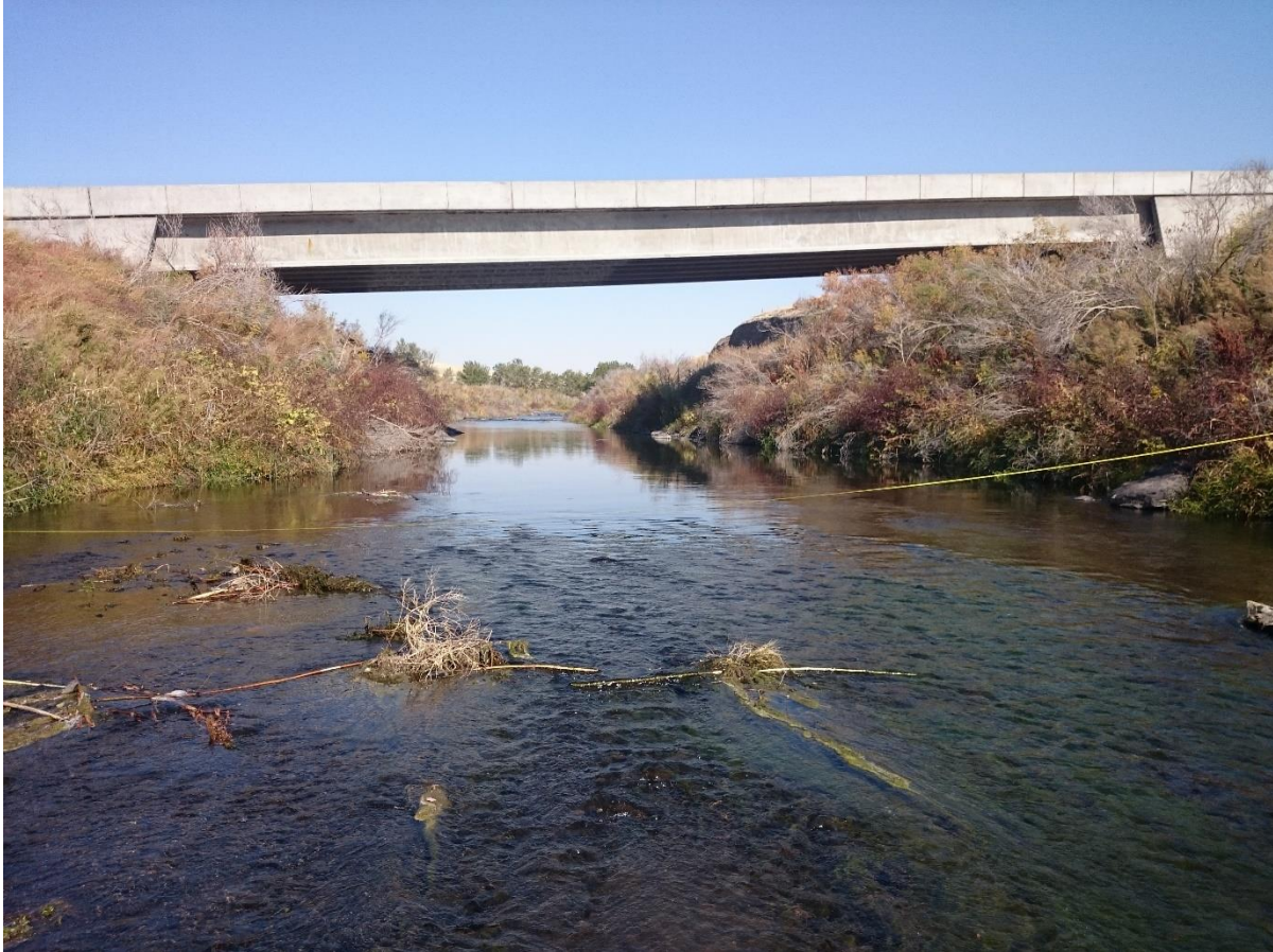
Touchet River at IW Sims Road Bridge
